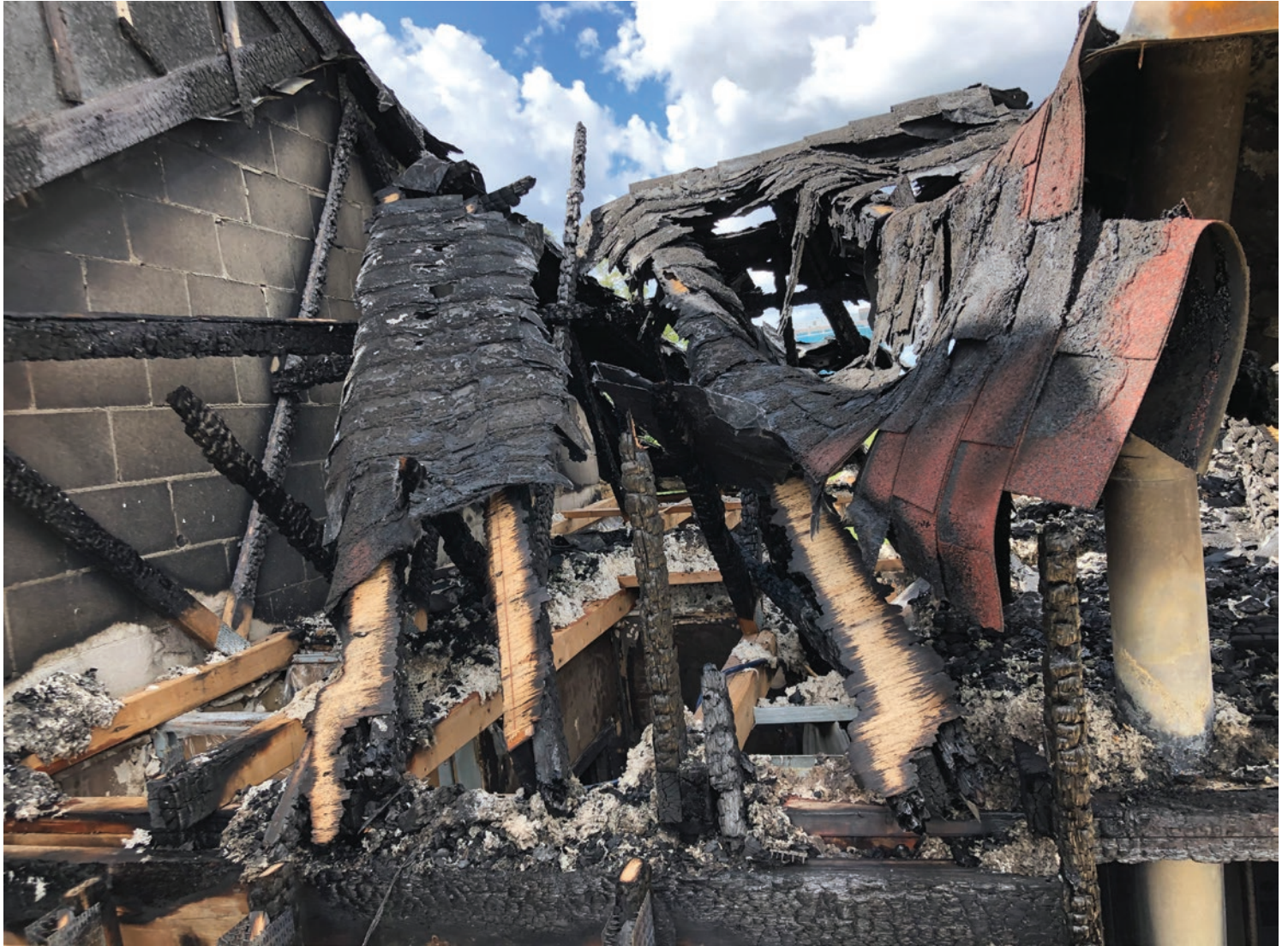
Concrete block fire separation between townhouse units (Photo credit: Y. Korany)
